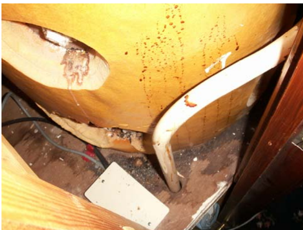
Water damage on a cylinder support shelf and visible leak from a corroding valve
