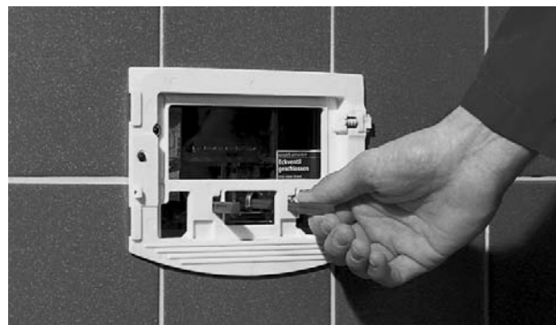
The push rods can be inserted quickly and accurately using the alignment shots
