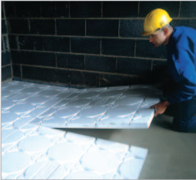
Installation of floating floor panels
