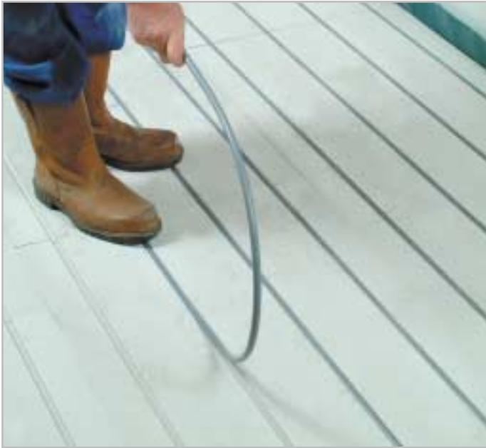
Pipe Installation with Overlay™
