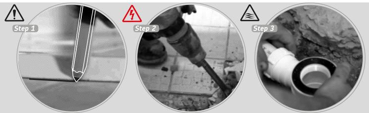
Secure in place and connect the waste outlet. Always clear away all excess adhesive. Support the bottom of the waste.
