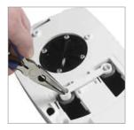
Lubricate the supply pipe ends using a silicone based lubricant and carefully slide the Aquastream Thermo unit onto the pipes whilst feeding the low voltage cable through the cable entry point. Secure the unit to the wall using the screws provided.
