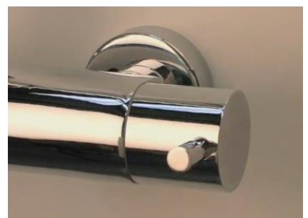
9. Re-fit the Temperature Handle Lever.
