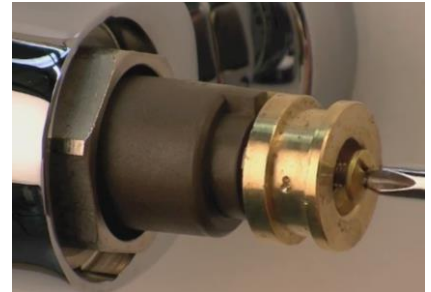
3. Using a X-head screwdriver, remove the Temperature Stop Lug.
