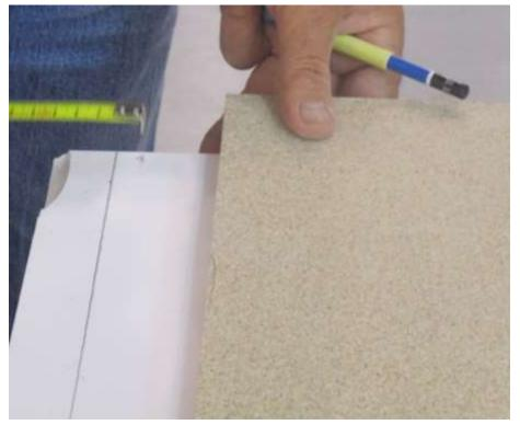
Measure the size of the grinder cap and bring the measurement back to the shower tray (offset from the cutting line)
