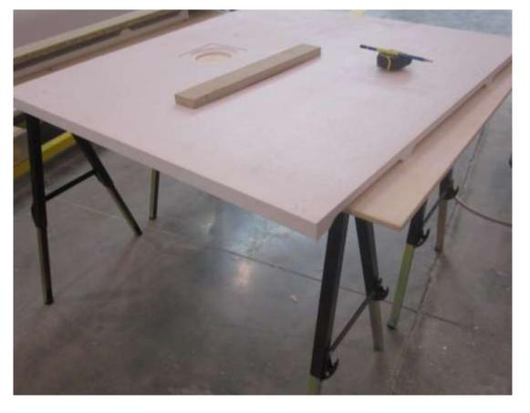
Trace the cut size directly on the surface of the shower tray using a panel that will then act as a spacer.
