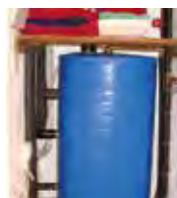
cold water tank installed in the loft
