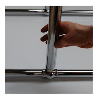
Now offer the rail up to the ceiling / wall and mark though the 3 hole on each wall/ceiling plate. Please ensure the orientation of the wall / ceiling plate is such that you can access the screw head to tighten this up with out the main rail interfering.
