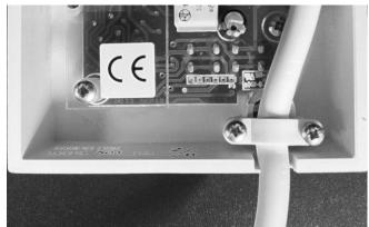
Carefully fit the control plate into the back box ensuring that no wires are trapped during the sitting process.
