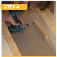
To allow support of the drain fitting aid and the drain body, construct a platform to suit the waste position in the tray. Using screws and glue, securley fix 50mm x 25mm timber battens to the floor joists then fix an 18mm marine plywood supporting base onto the battens.
