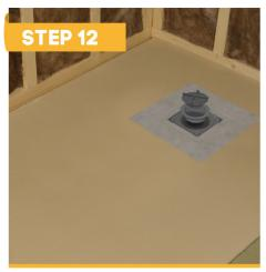
Using the securing tool supplied with the drain, screw the threaded waste collar into the drain body before the adhesive hardens. Care must be taken to fully tighten the assembly to ensure a watertight seal is achieved. The securing tool should be left within the drain body at this stage to protect against debris falling into the drian during tiling and grouting.
