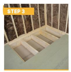
With the tray position marked out, the floorboards can now be removed. Following the markings on the floor cut through the floorboards using an electric saw. Check the saw blade is set to the correct depth to avoid damage to the existing joists or any pipework/electrical cables which may be concealed below.
