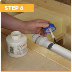
Once the platform is installed, place the drain fitting aid and drain body into position. Using 1 1/2" ABS fittings, fix the waste pipe into the drain body using a solvent weld. Its is important at this stage to check for any leaks, as you may not be able to return to this assembly at a later date.
