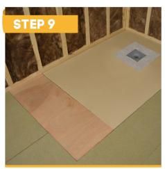
Now check the alignment of the drain body and the drain aperture in the tray. Make sure they are perfectly aligned and if necessary adjust accordingly. The tray should now fit onto the newly created platform but sit slightly proud of the remaining floor area. Exess floorboards may have been removed back to the next joist centre. This can be backfilled using marine plywood at the necessary thickness to suit.
