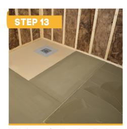
With the tray fxed into the adhesive, the surrounding floor area can now be overlaid with Tile Backer Boards. It is very important that the existing floorboards must be securley fastened to the joists using suitable screws. If previously ficed with nails, additional screws should still be used.
