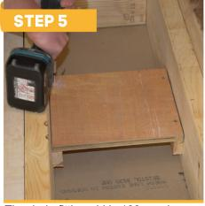
The drain fitting aid is 100mm deep and it is important when setting out the supporting platform to allow for the thickness of the fitting aid to finish flush with the top of the floor joists.
