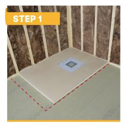
Clear the working area from loose debris and grease. Place the Underlay Plus onto floorboards to allow marking out of the tray perimeter onto the floor. When setting out the position of the tray it is important to remove the floorboards past the edge of the tray and back to the centre of the next joist. Check that the position of the drain does not conflict with joists below the floorboards.
