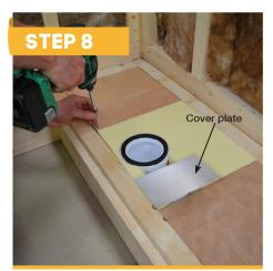
With the battens secured, an 18mm thick plywood support platform must be placed between the joists to support the entire base of the tray. The 18mm plywood should be screw fixed to the 50mm x 25mm timber battens and should finish flush with the top of the floor joists.
