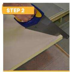
If the drain conflicts with a joist or other obstruction, the tray side can be trimmed to alter the drain position.
