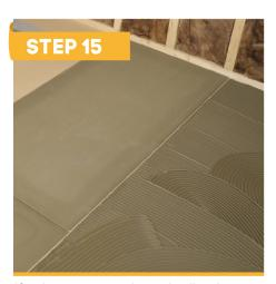
If using a cement based adhesive to fix the Tile Backer Boards, the existing floor must be primed using a suitable floor primer. Apply a solid bed of adhesive using a thick notched trowel and firm down the boards into the bed
