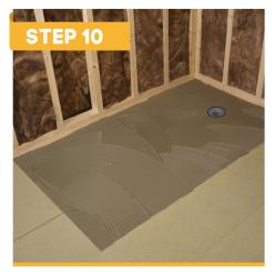
The Underlay Plus can now be fixed into place using a good quality, cement based rapid setting flexible tile adhesive. Apply the adhesive with a thick bed notched trowel to the area where the tray is to be placed. Make sure adhesive is applied over the stainless steel cover plate. When applying the adhesive around the drain it is important to leave a 10mm gap between the adhesive and the main rubber seal of the drain body.
