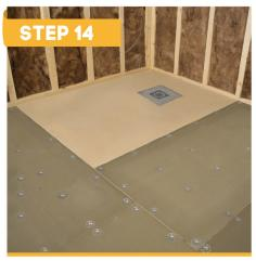
If the Tile Backer Boards are to be fixed using a dry fix method, washers should be positioned at approx. 200mm centres. It is important to use the correct length of screw to avoid penetration of the floorboards when fixing in place.
