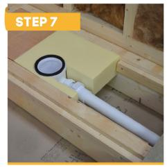
With the drain body and waste route now installed and tested, a structural platform to support the tray can be fitted. The Underlay Plus is not designed to span joists, therefore it is essential that the entire base of the tray is supported by a structurrally stable surface. This is achived by securley fixing 50mm x 25mm battens set 18mm below the top of the floor joists. The battens should be fixed using glue and screws to the supporting joists.
