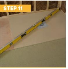
With care place the tray into the adhesive. Make sure the rubber seal of the drain remains firmly seated on the drain body. Apply moderate pressure to the entire surface of the tray and around the drain aperture, making sure there are no hollow spots beneath the tray.
